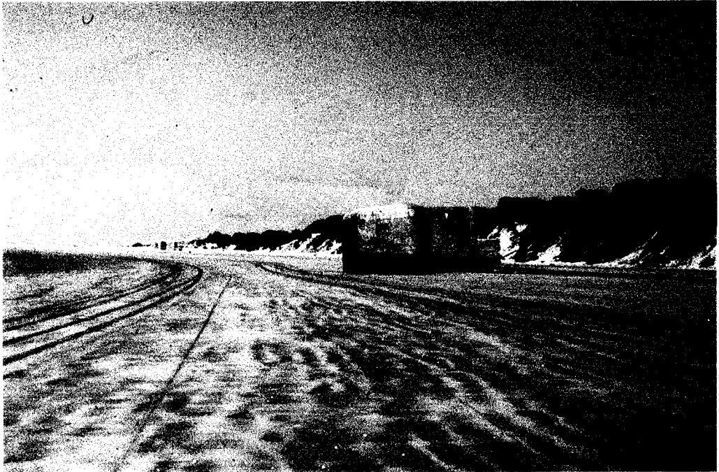
Figure 4: Bunker initially installed upon former dune ridges, today fallen on the intertidal zone of Malandar Beach (Doñana National Park).
